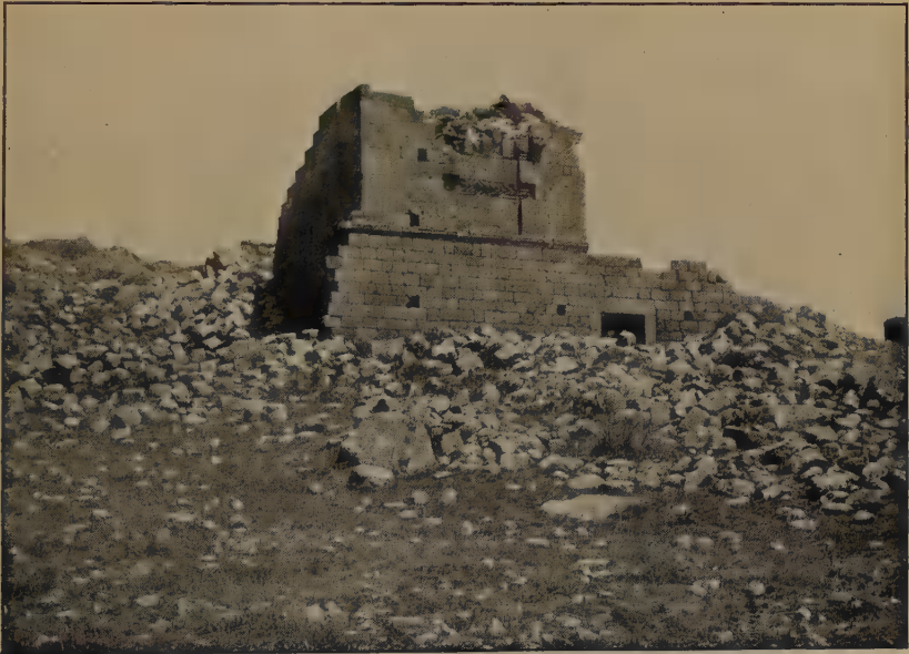
Part of a Monastery above Bin-Bir-Kilisse, showing short zones of brick used as ornament in a stone building. To face p. 124. See p. 161.
